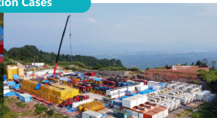
A block in Weiyuan use the well gas to power the electrical fracturing pump unit
