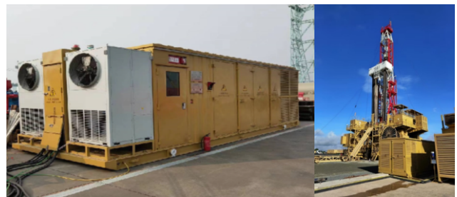
A battery energy storage system (BESS) with power management system (PMS) powers the rig on a Total drilling platform Achieve energy efficiency optimization control and reduce carbon emissions
